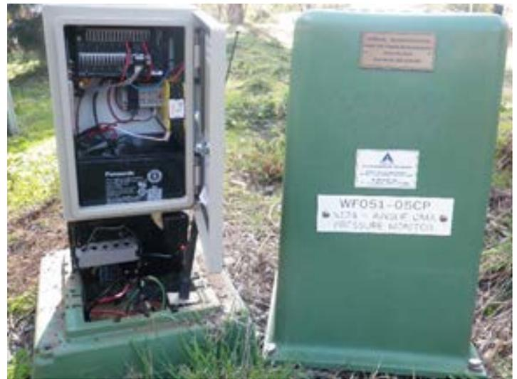
Figure 1. Installed pressure monitoring station
