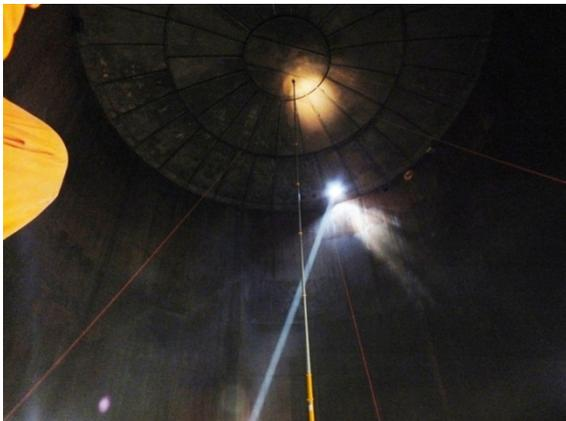
Figure 3: Telescopic pole fully extended, to the top of the tank roof
