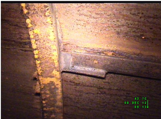
Figure 5: Image of side wall showing mild corrosion
