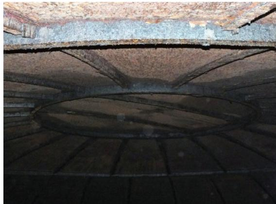
Figure 4: Image of roof structure, showing mild corrosion
