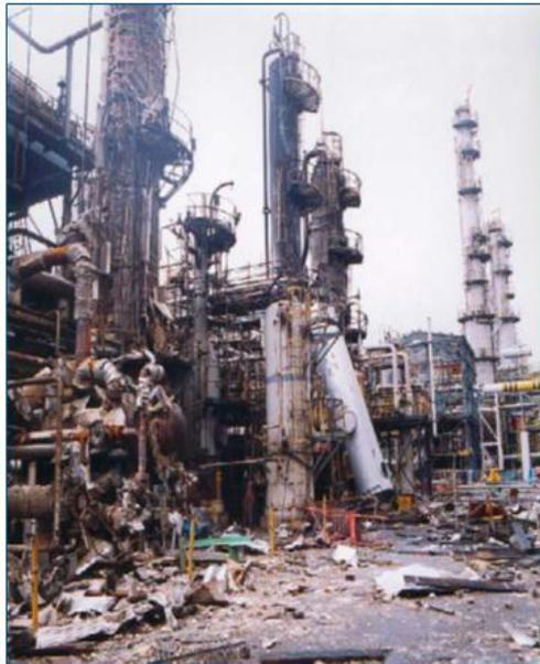
Fig 1. Damage caused by rupture of a pipe elbow at the Humber Refinery, UK 2001.
