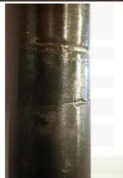
CuNi tube - ammonia attack at baffle location
