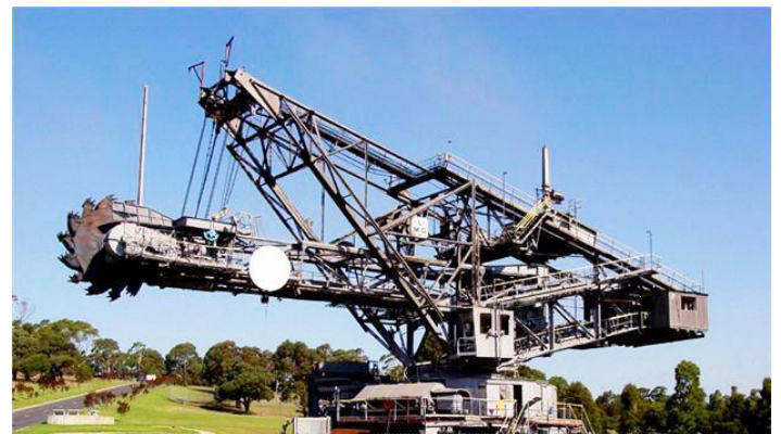
Figure 1 – A Bucket Wheel Reclaimer, for which ALS provides inspection of Bucket Wheel Shafts, Boom Pivots and Crawler Beam Axles
