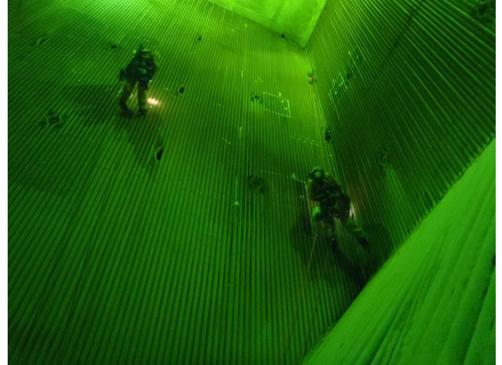
Figure 2 – Two man team performing internal rope access
