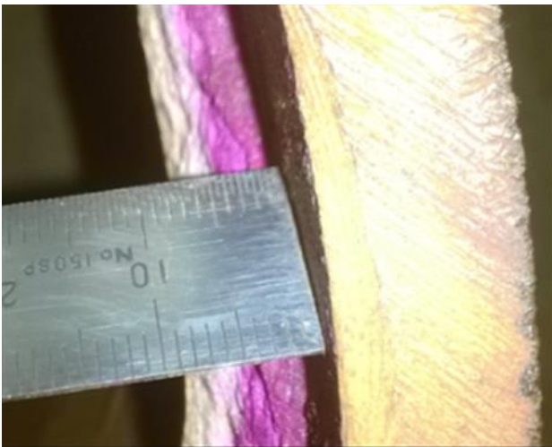
Figure 3 – Measurement of the concrete lining showing loss of alkalinity
