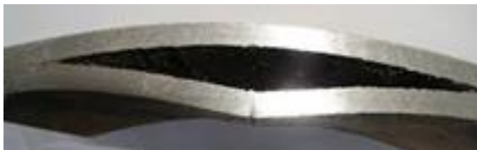
Figure 1: H 2 blistering in steel tank plate due to internal corrosion
